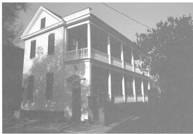
Fig. 10. Charleston, SC. Traditional dwelling type (narrow street frontage) provides ventilation. shaded portico facing interior courtyard garden for sun tempering and cross-ventilation
